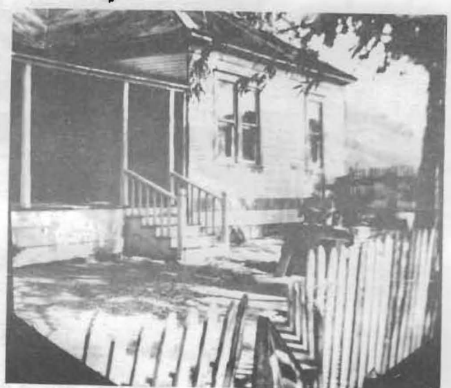
New house in Collier Canyon.
