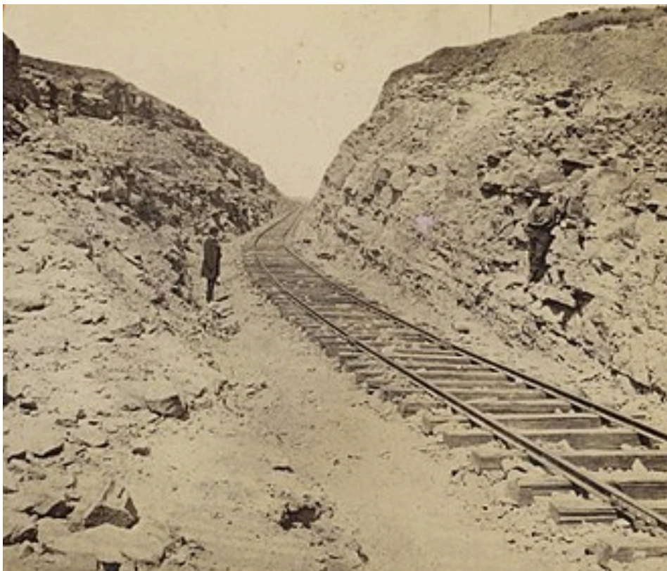
Above: The Deep Cut: Approximately 100,000 cubic yards were removed by hand with horse and cart. Photo courtesy of DeGolyer Library, Southern Methodist University.
